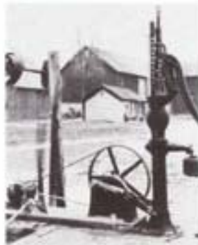
One of the first uses for electricity on South Texas farms in the 1920s was for pumping water. Note the wire leading into the insulator attached to the wooden plank.
